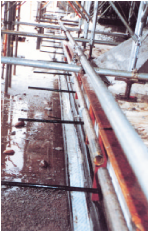
Condition of the waterstop after the primary concrete is poured.
