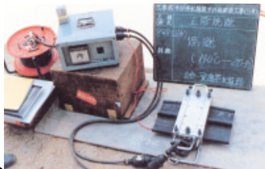
On-site jointing of waterstop using an Joint Mold ▶
