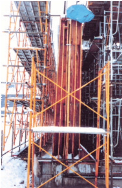
Waterstop firmly interposed waterstop between the forms.
