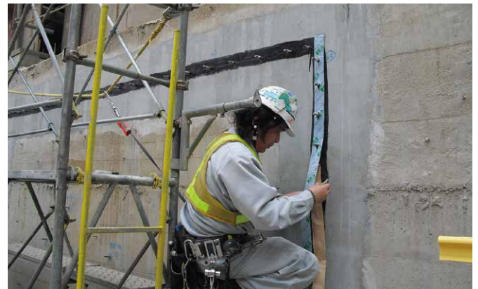
1. Span seal installation
