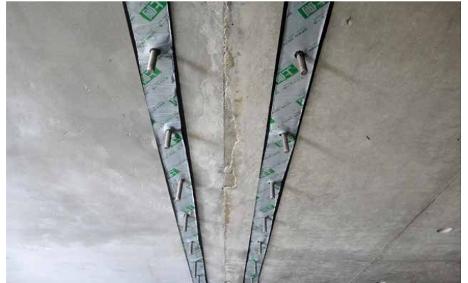
5. Span Seal installation
