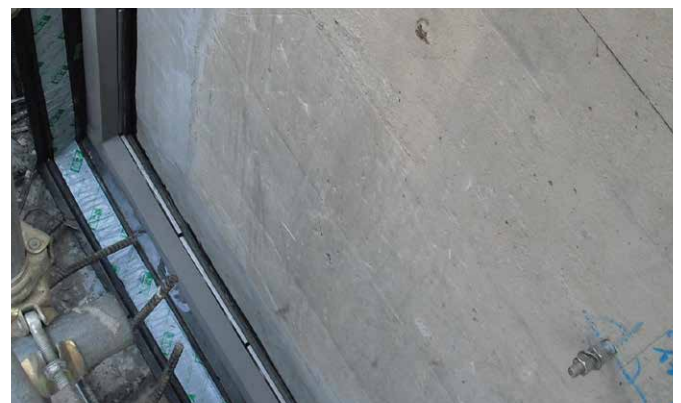
4. Expansion joint filler installation
