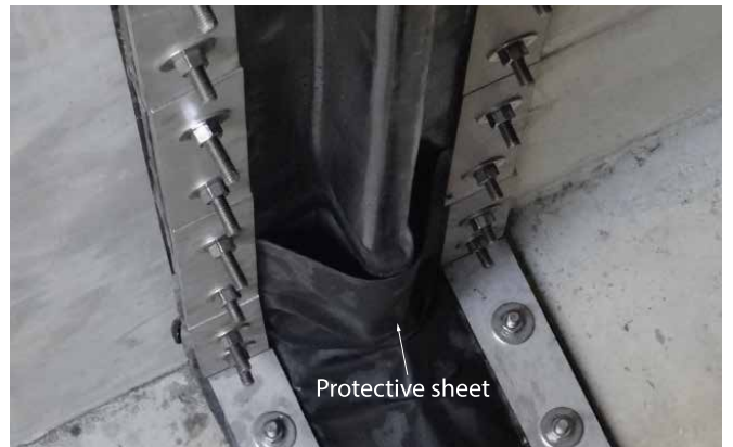
7. Protective sheet installation
