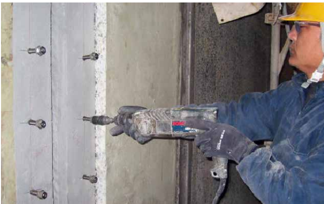
3. Anchor installation
